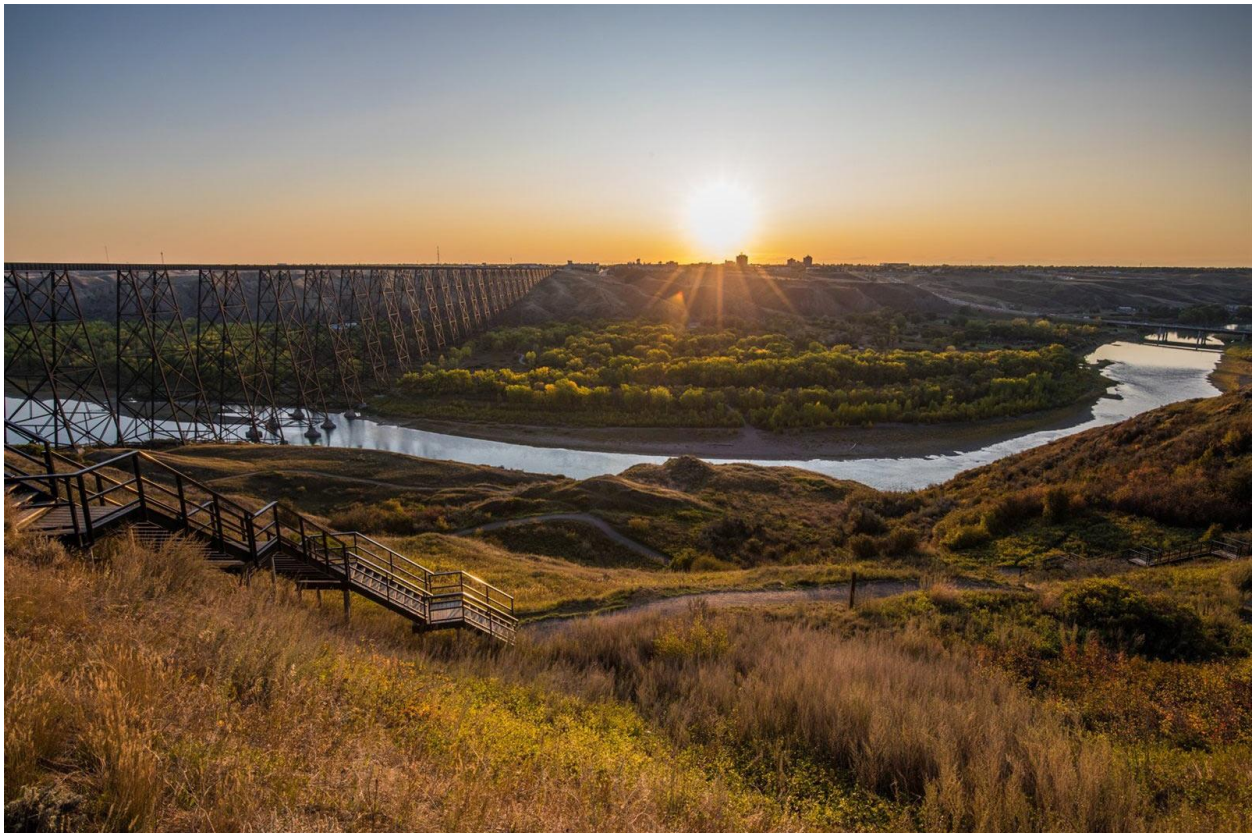
The Leth Bridge over the Old Man
